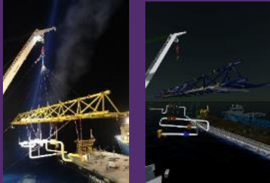
Kaombo spool installation (simulation is on the right)
