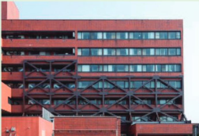
An example of a seismic retrofitting: External steel frame
