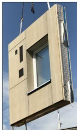
Figure 8: Functional sample of a prefabricated wooden façade with integrated outdoor unit of the heating-ventilation-heat pump. Image source: [21].
