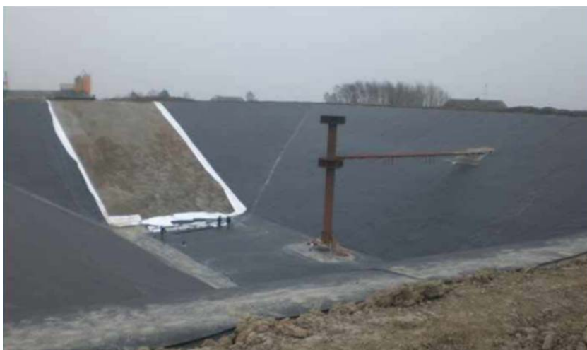
Figure 3 : "Water Pit Storage" en construction [3]
